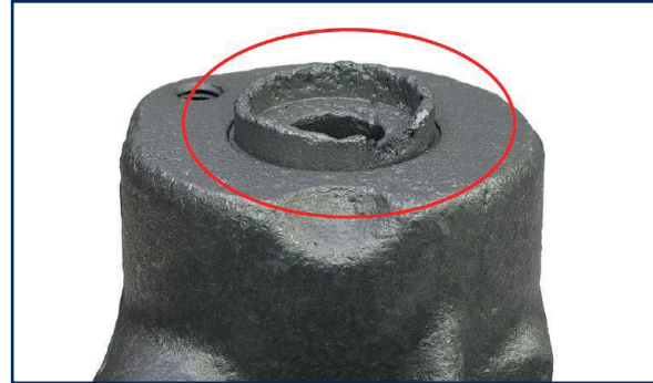
The inner cylindrical part has been corroded and is broken.
